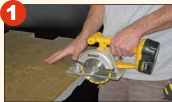
Cut panel to length with standard saw.
