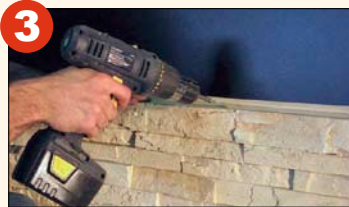
Fasten panel to wall at flange with screws.
