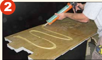
Apply polyurethane adhesive to panel back.
