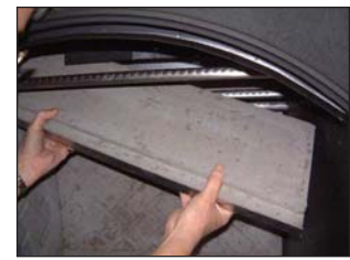
Tilt Baffle downward towards front of fireplace FIGURE 8
