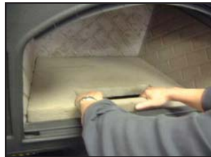
FIGURE 4 Bottom and Front Refractory
