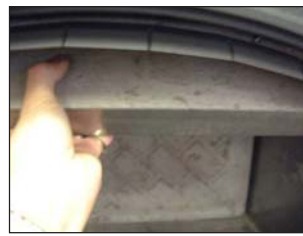
Tilt Baffle downward toward the front of fireplace FIGURE 7
