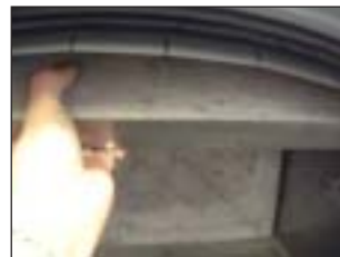
Tilt Baffle downward toward the front of fireplace FIGURE 8b
