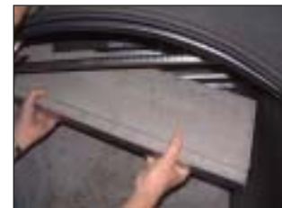
Tilt Baffle downward towards front of fireplace FIGURE 8c
