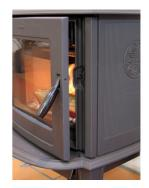
8. When the primary air supply is opened all the way and the door is closed, the new fuel will ignite in a few minutes.
