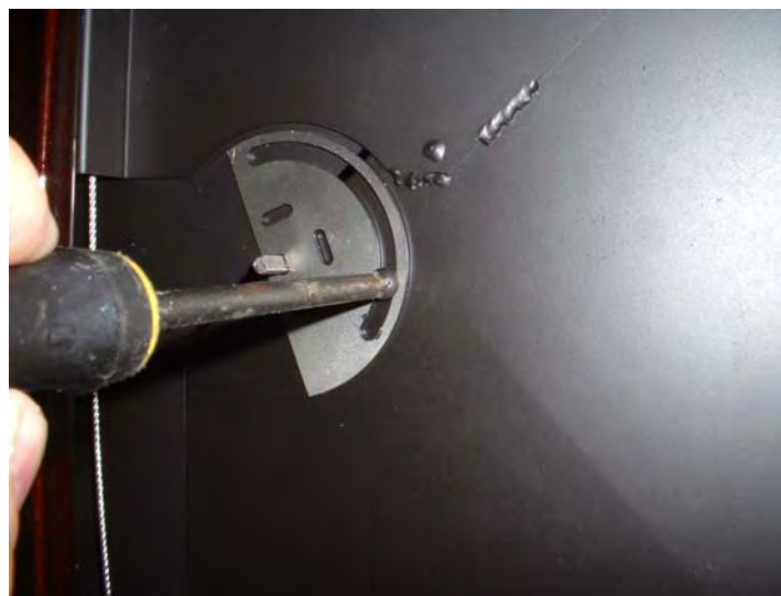
Photo 14: Restrictor Fully Opened (no restriction)
