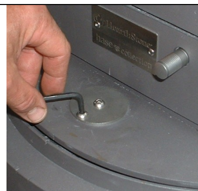
Figure 7 - Tighten Mounting Screw
