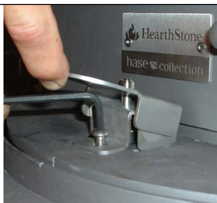
Figure 4 - Remove Mounting Screw
