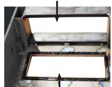
BYPASS DOOR OPENING
